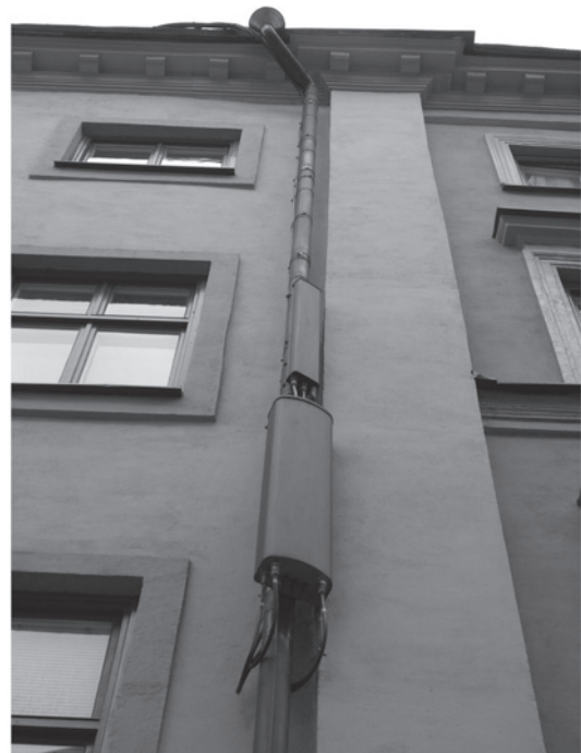
Figure 12. Stockholm Old Town measurement location with a relatively high radiofrequency radiation level, due to a mobile telephony base station antenna positioned at a low height and targeted towards the square.
